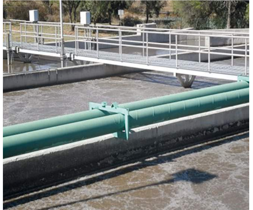
Reactor aerobio
