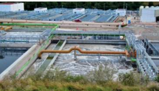
Reactor aerobio
