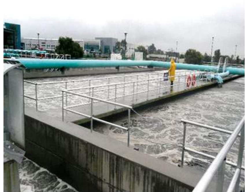
Reactor aerobio
