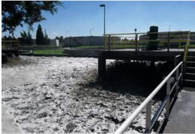
Reactor aerobio
