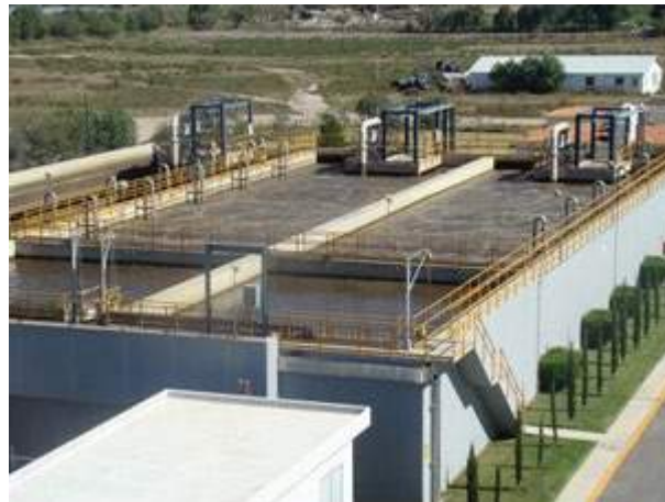
Reactor aerobio
