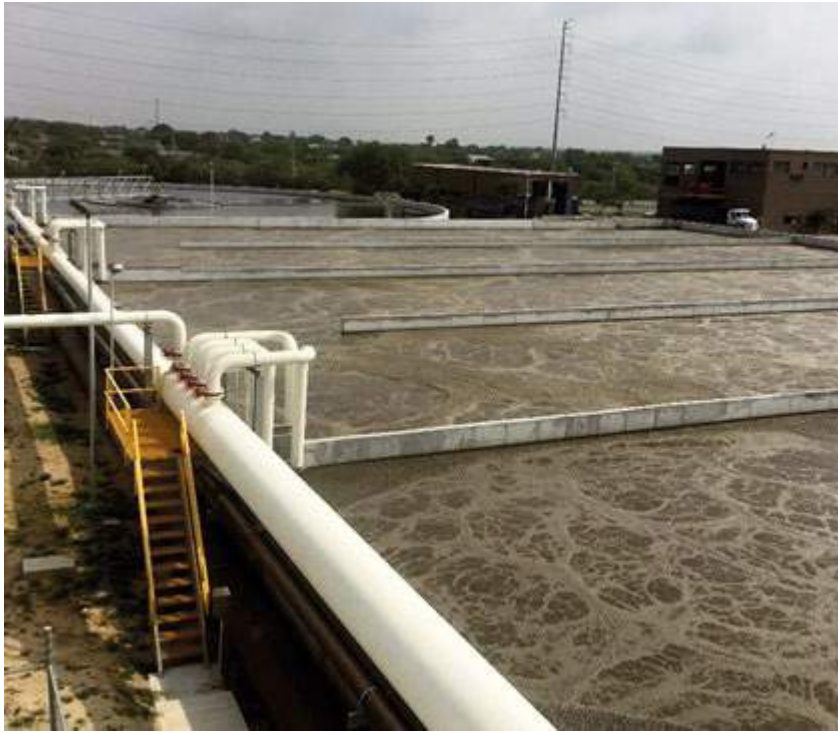
Reactor aerobio
