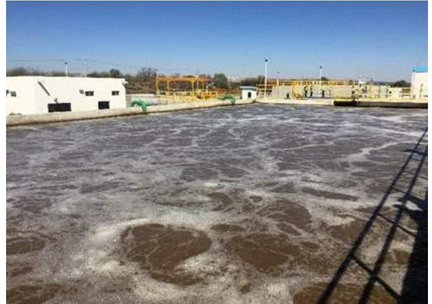
Reactor aerobio
