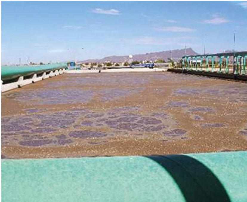
Reactor aerobio
