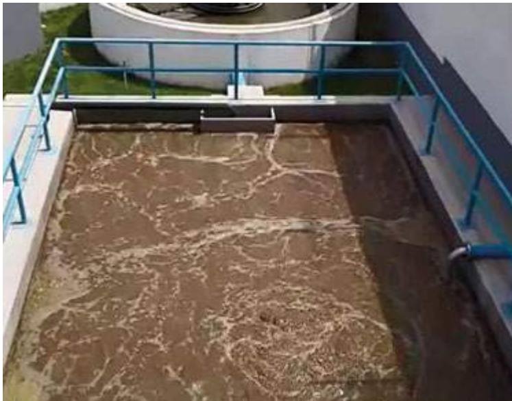
Reactor aerobio
