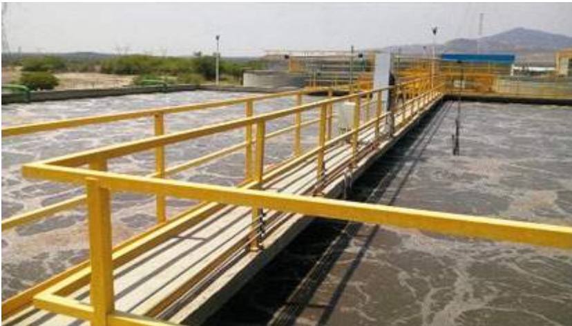
Reactor aerobio
