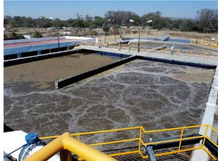
Reactor aerobio
