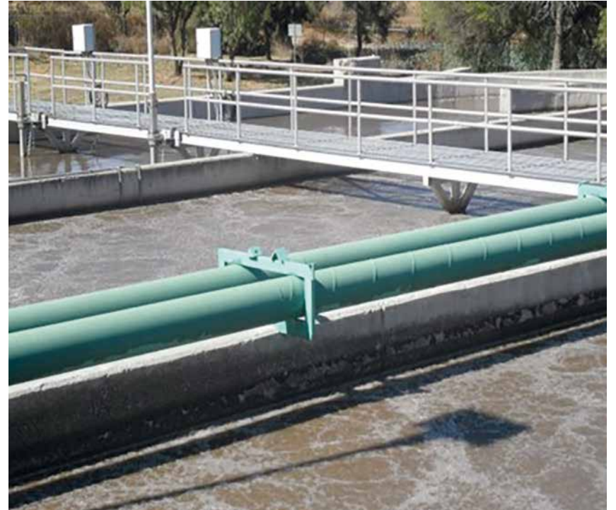
Reactor aerobio
