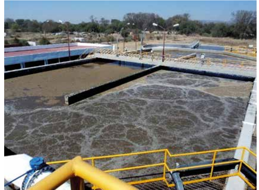
Reactor aerobio
