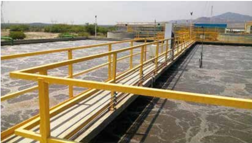
Reactor aerobio
