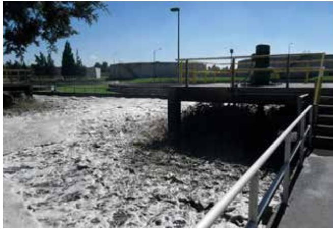
Reactor aerobio
