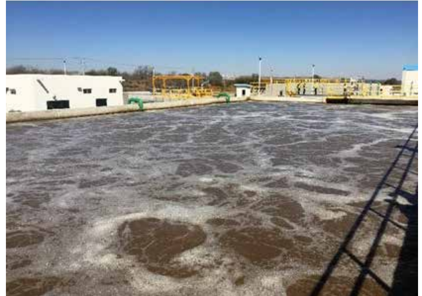
Reactor aerobio
