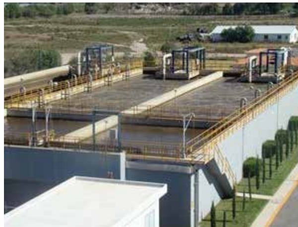
Reactor aerobio
