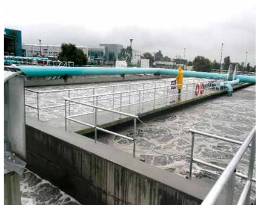
Reactor aerobio
