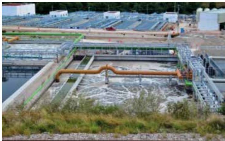
Reactor aerobio
