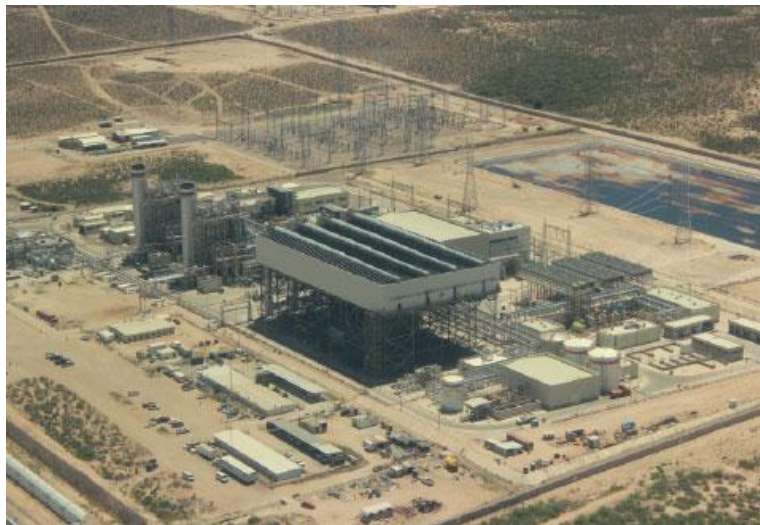
Figure 2.43. Agua Prieta II combined cycle power station. Source: (SENER, 2016)
