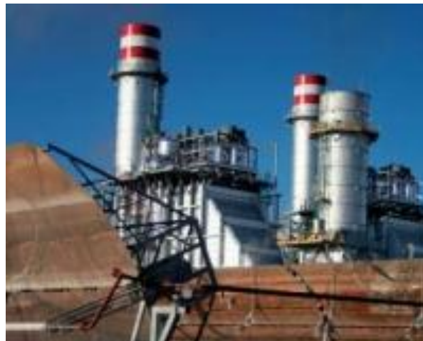
Figure 2.46. Ain Beni Mathar power plant. Source: (ABENGOA, 2019)
