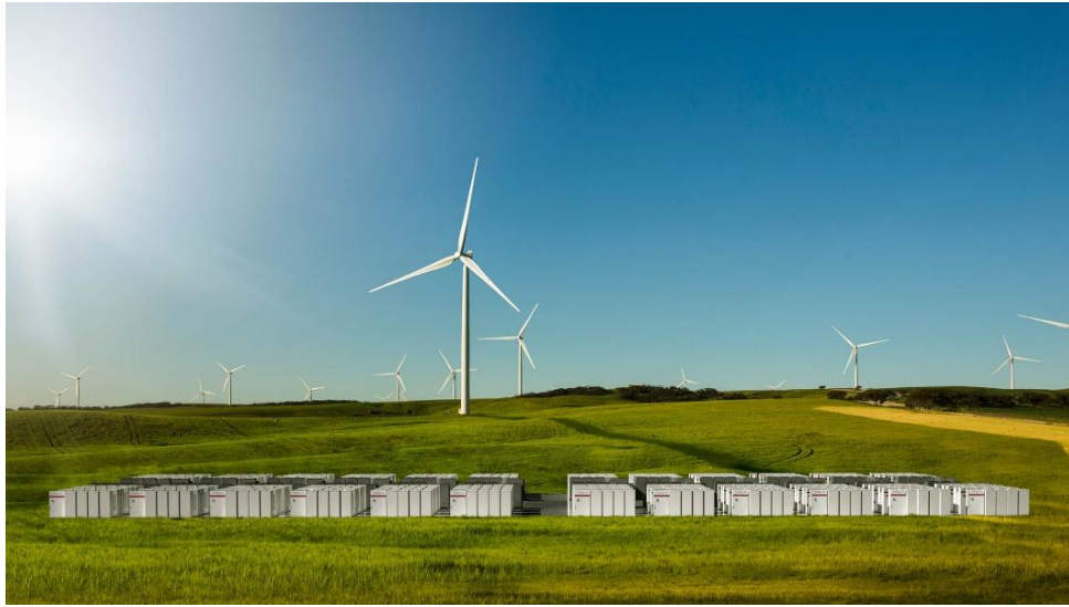
Figure 2.15. Render of Tesla Powerpack System to be paired Neoen's Hornsdale Wind Farm near Jamestown, South Australia. Source: (Tesla, 2017)
