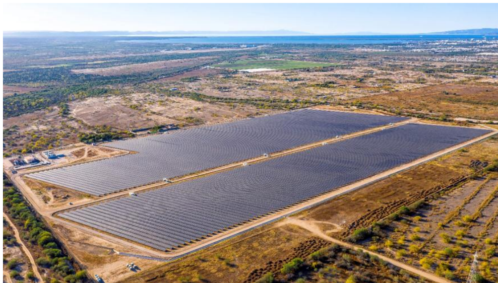
Figure 2.18. Solar plant Aura III in La Paz, Mexico. Source: (pv magazine, 2019)
