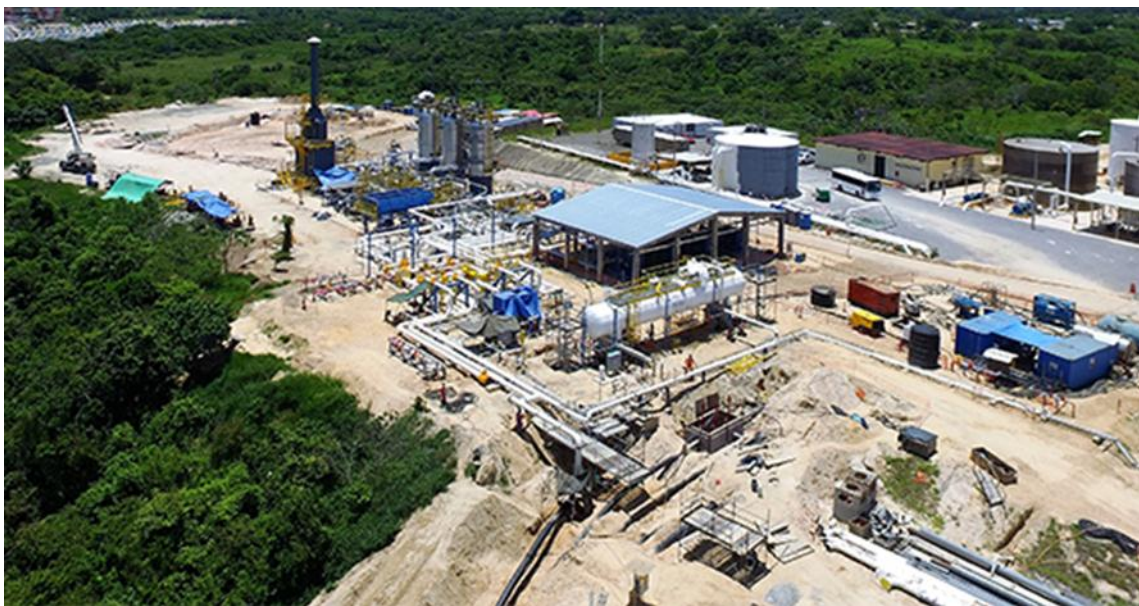
Figure 1.16. Surface infrastructure of the underground CYDSA-PEMEX salt-cave based LP gas storage facility in Veracruz Mexico. Source: (CYDSA, 2020).
