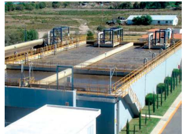
Reactor aerobio
