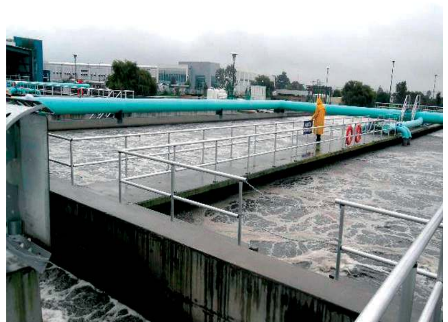
Reactor aerobio
