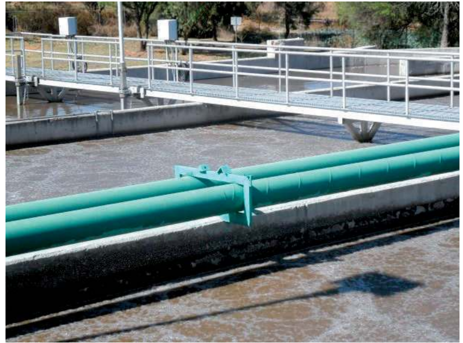
Reactor aerobio
