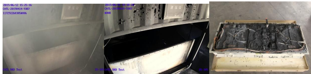
d) released fire extinguishing agent e) no burnback f) battery residues
