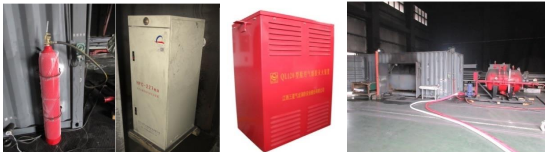
a)Carbon dioxide b)Heptafluoropropane c)Aerosol d)Pressure water mist, low-expansion foam
