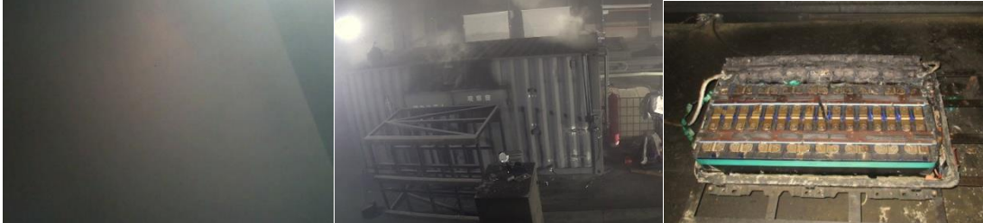
d) released fire extinguishing agent e) no burnback f) battery residues
