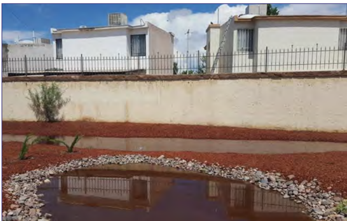
Passive rainwater harvesting systems at the park.
