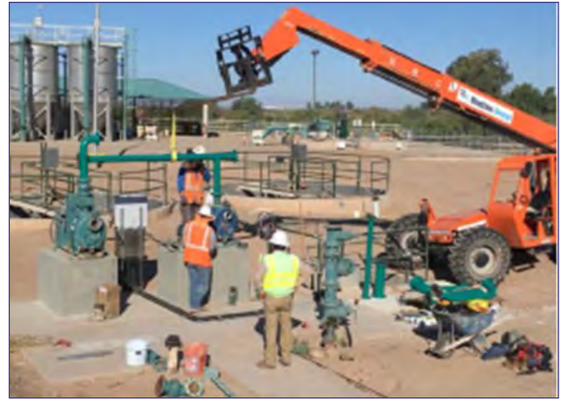
Building a stormwater pump station.
