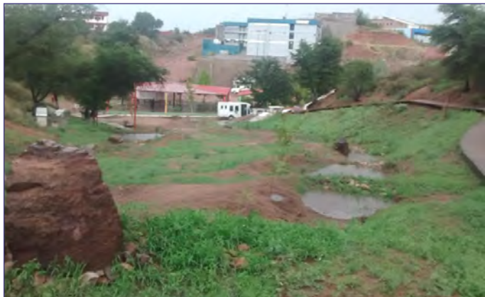
Rain park designed to harvest rainfall and prevent flood events.
