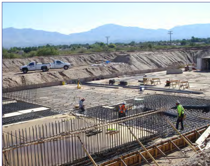
Construction activities for the new Sunland Park treatment plant.
