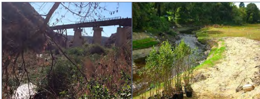
A section of the Tijuana River basin before the start of the work and another section after the restoration activities.
