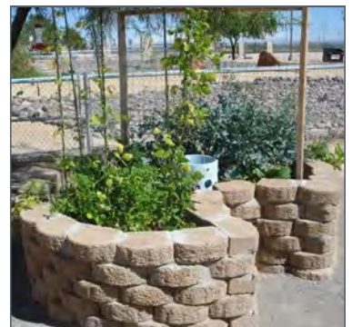
One of the keyhole gardens constructed.
