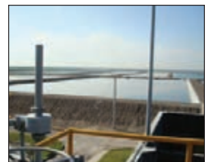
Matamoros West Wastewater Treatment Plant (WWTP): A lagoon system and the first WWTP for the City of Matamoros.
