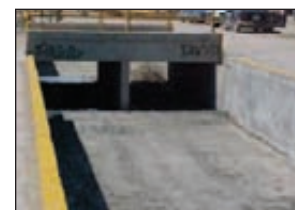
Canal after clean-up.
