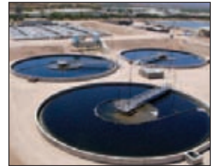
Nogales Waste Water Treatment Plant.
