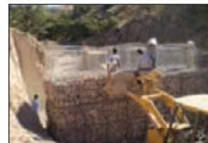
Stormwater Detention Structure.
