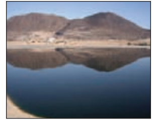
Las Arenitas Waste Water Treatment Plant.
