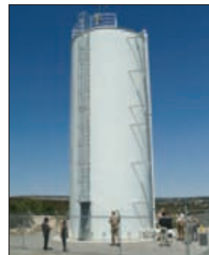
New Water Storage Tank to Serve Campo Band of Mission Indians.
