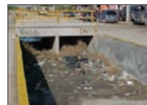
Canal before clean-up.
