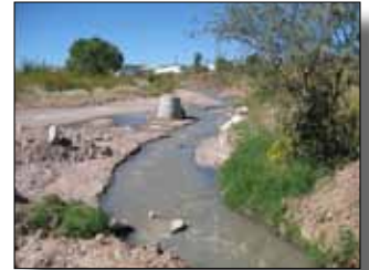
Stream gauge on the Nogales Wash providing Internet-accessible, real-time flow data.
