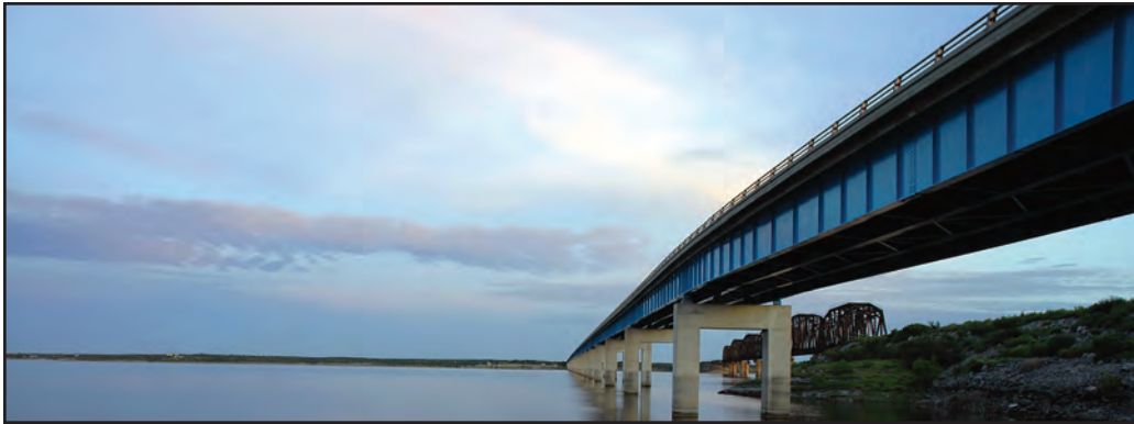
A bridge over Amistad Dam, upstream from the border sister cities of Del Rio-Ciudad Acuña, serves as an example of important infrastructure for cross-border emergency preparedness and response.
