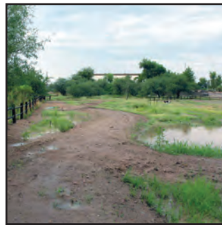
A raised, meandering path acts as a berm to retain storm water runoff near the Santa Cruz River in southern Arizona.
