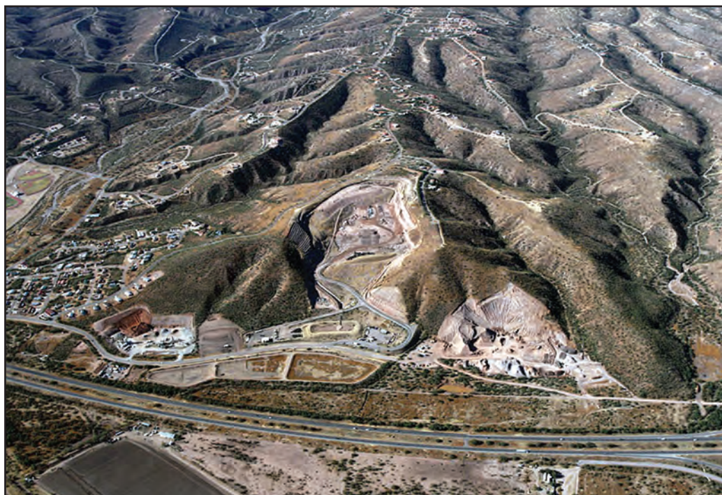
Landfill gases from the Río Rico Landfill, a 60-acre facility located 14 miles north of the U.S.-Mexico border, are deemed sufficient to generate electricity for 30 years.
